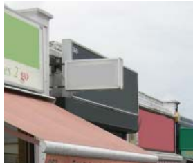
Fascia signs that project out and block the view to separating pilasters
