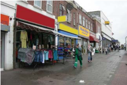
Facia signage breaks up the continuity of the cornice
